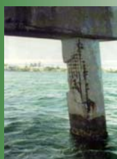
Bridge piers subjected to corrosion
